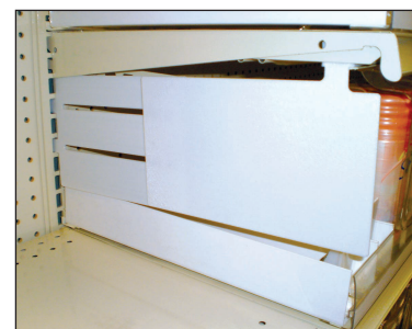
Left Metal End Panel and Extender installation is complete.
